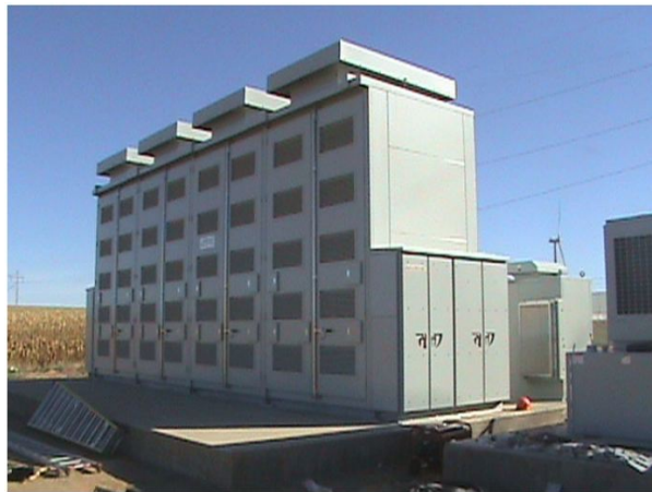
Xcel Wind-to-Battery Project Luverne, MN 2008 1,000 kW Sodium Sulfur Duration: 7 hour at 1MW
