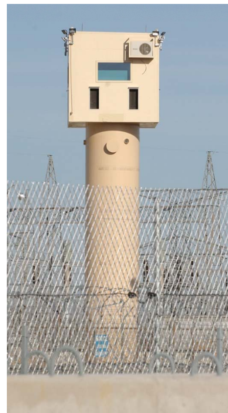
New security tower at the Clinton nuclear plant
